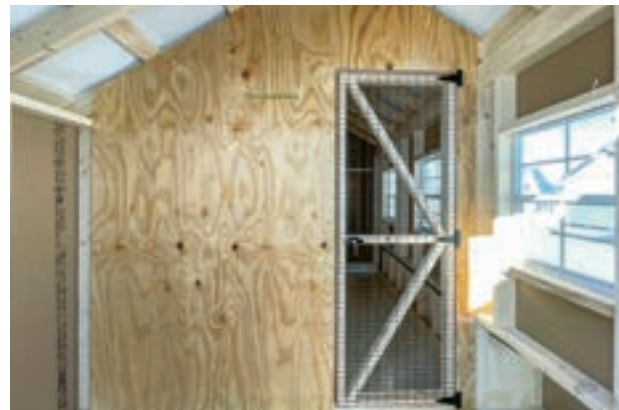
Solid plywood wall with screened door
