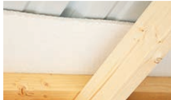
Insulated Ceiling Standard on Metal Roof option
